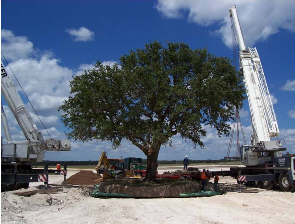
Tree Placed Before Construction of Entry Drive
